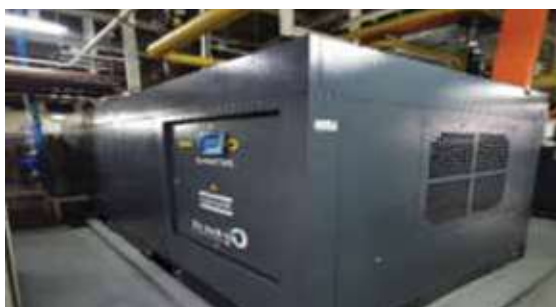
High efficiency 500kW centrifugal compressor
