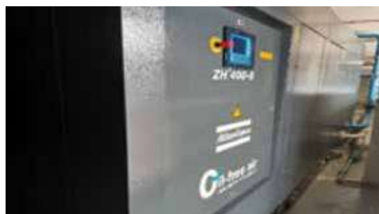
High efficiency 400kW centrifugal compressor
